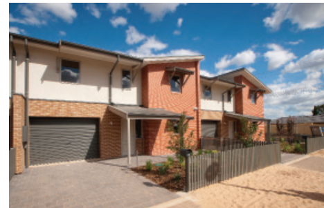
Two storey housing at Playford North
