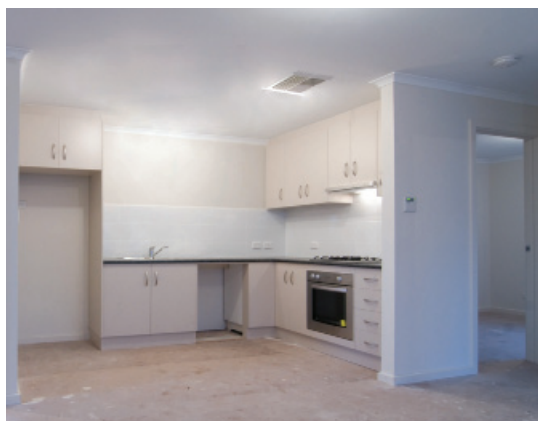
Compact kitchen fit out in a 2 bedroom mews dwelling. Showing overhead cupboards including rangehood, fitted under bench oven and cooktop, fridge space and dishwasher space
