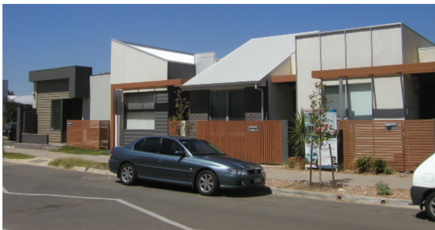
Narrow lot affordable row housing at Mawson Lakes
