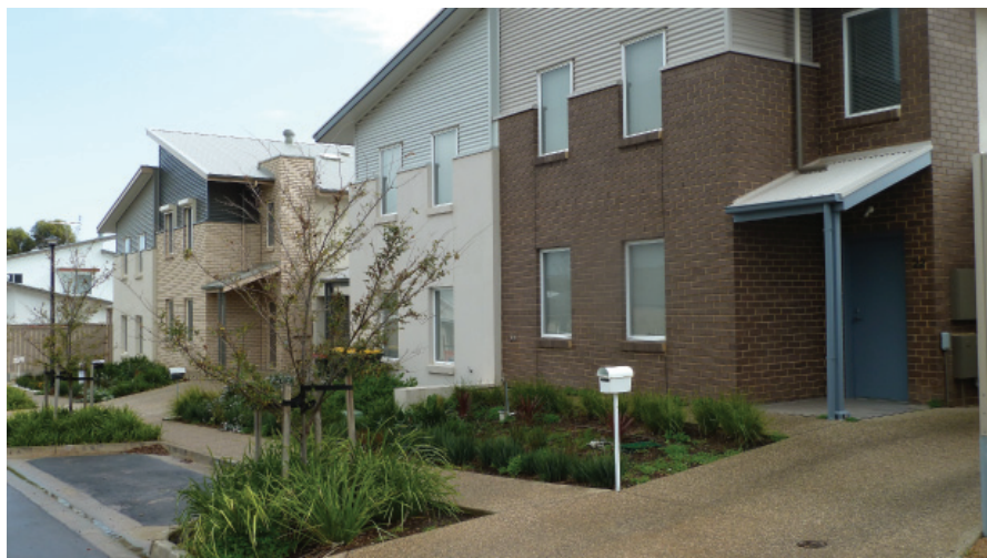
Two storey terrace housing at “Inspire” in Noarlunga Centre
