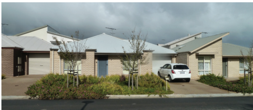
Single storey dwellings at “Inspire” in Noarlunga Centre
